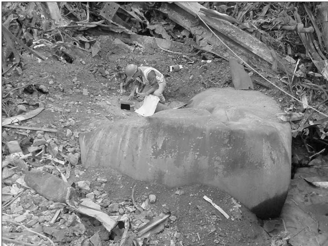
DEC inspector on top of a 20,000 gallon tank that was crushed by the partial collapse of a building.
