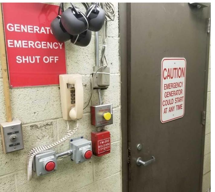
Manual Stop Emergency Shut Off switch is just outside door of generator room and properly labeled.
