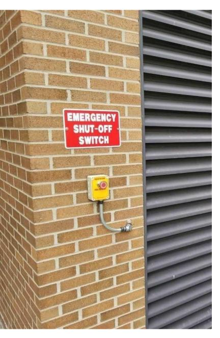
Emergency Shut Off switch for this outdoor generator is properly labeled on nearby outdoor wall.
