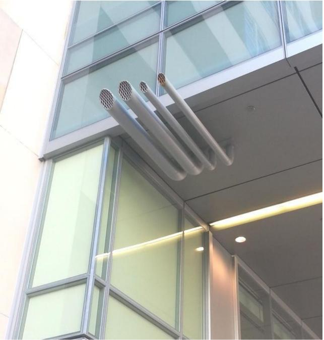
This is <u>not</u> how the normal and emergency vents should discharge from the basement day tank. There are hidden traps in inaccessible ceilings inside building.
