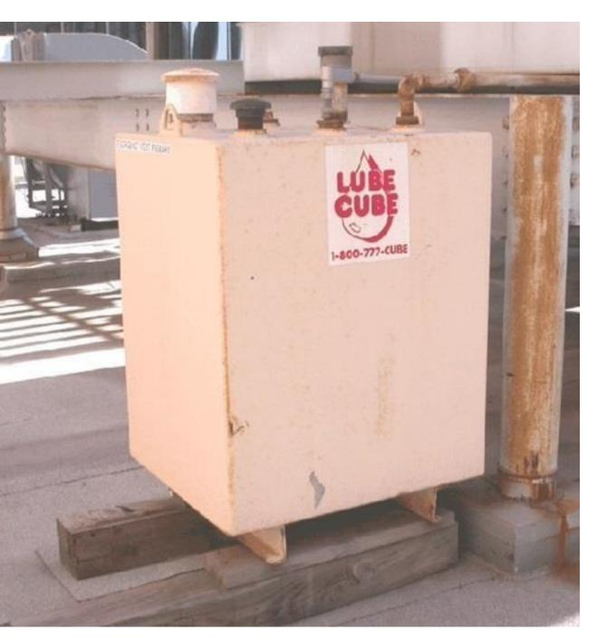
Don't forget to look on roofs for day tanks. Note wooden supports and other code violations. This tank has only "fill" control. When float switch got stuck, pump overfilled it with several thousand gallons of No. 2 diesel.
