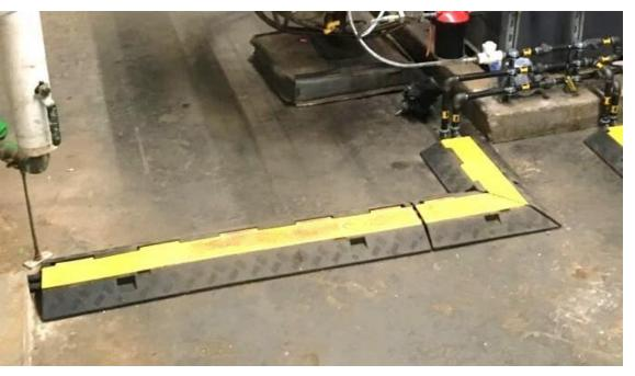
There are many excellent and cost-effective ways to keep sidewalk and aisleway traffic (including movement of equipment) from damaging fuel piping.
