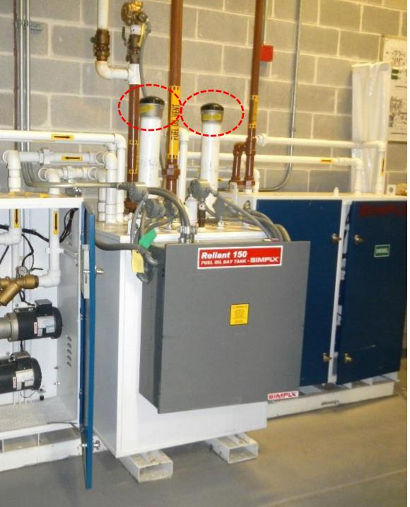
Here the day tank **Emergency Vents** highlighted in red discharge directly into the building. Any problem with the filling will result in fuel flowing out the E-vents and down the corridor
