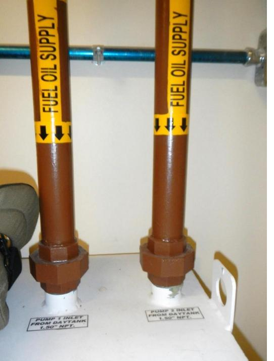
ASME B31 Power Piping means Schedule 40 steel. This includes all fittings, elbows, tees and other piping components.
