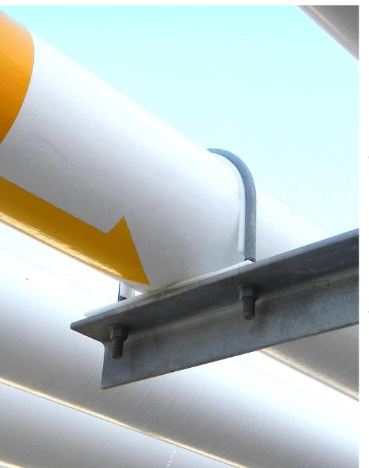
MSS-SP-69 supports are designed to minimize crevic corrosion and faying damag to pipes. Note the white pads beneath U-bolt and between the bottom of the pipe and the angle iron. Thi spacing allows inspection of the pipe by removal of the support as well as replacement of the pads.
