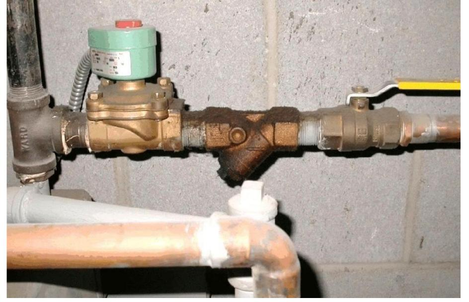
Regardless how often it happens, you cannot use low melting point piping and valving components inside a building for a day tank connected to a diesel generator.
