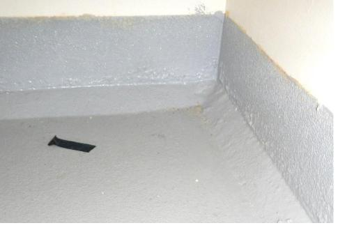
Must have liquid-tight floor in room with day tank. Floor must seal to the walls as shown at the left.
