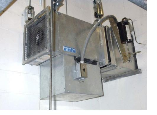
HVAC system in room with AST requires auto-closing fire dampeners on wall penetrations which are missing in top photo.
