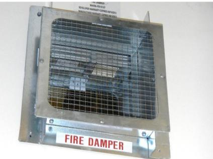
Bottom photo shows auto-closing dampers in place at wall penetration of a day tank room.
