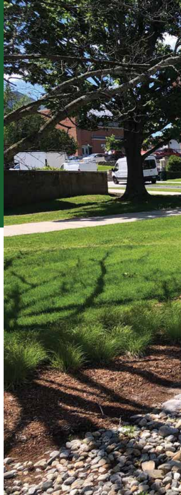
Above, a bioretention swale on the University of Connecticut's Storrs campus. The swale removes pollutants from road runoff and promotes infiltration.
