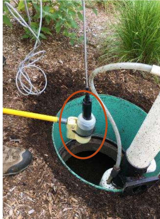
Collect final effluent sample
