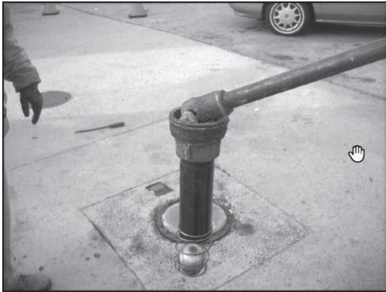
FIGURE 7-3. To avoid damage when removing or reinstalling the ball float, use an extractor tool recommended by the ball float manufacturer.
