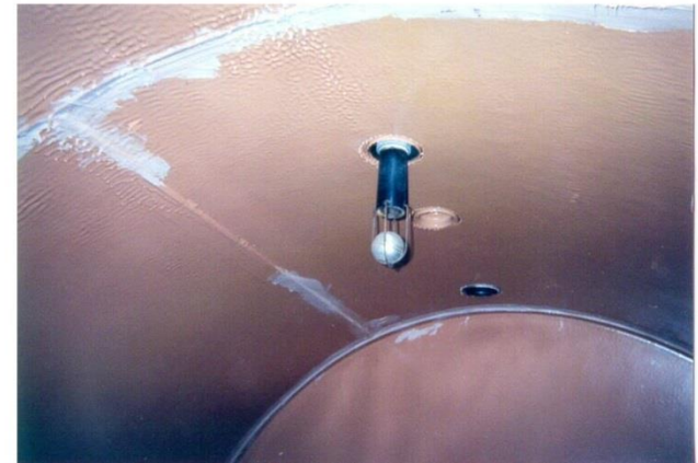
Ball float valve as seen from inside the tank
