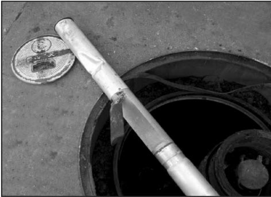
FIGURE 7-1. Check the drop tube and flapper for damage. Make sure that the flapper moves freely and will move into the product flow path.
