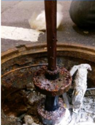
F1. - ATG Floats w Corrosion Products
