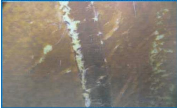
92 Octane UST – breakdown observed during pre-blast inspection
