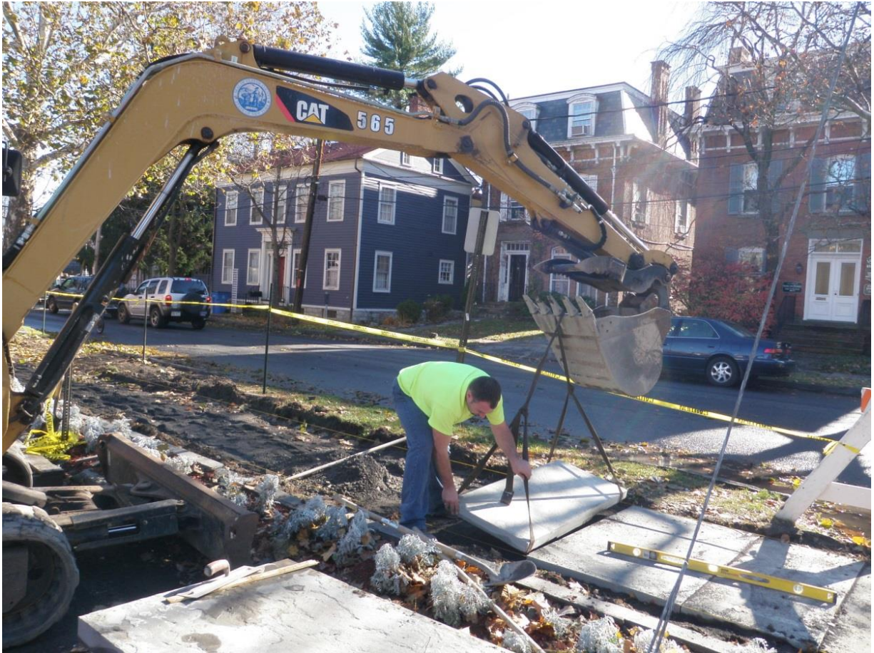
New bluestone sidewalk being laid down along Pearl Street
