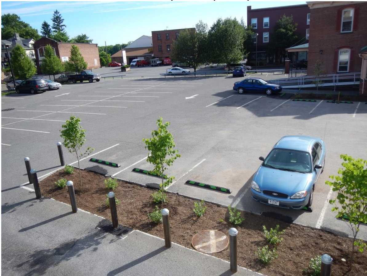
Installed curb-stops and un-painted posts
