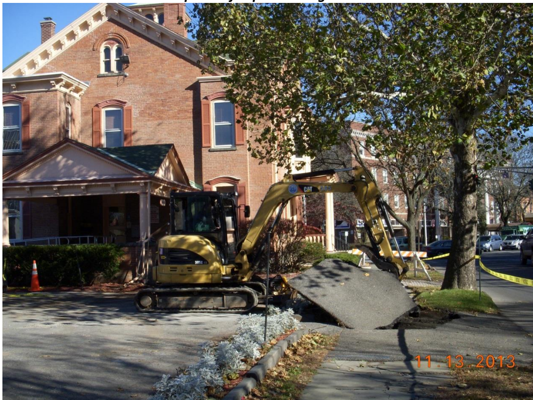
First piece of asphalt being removed
