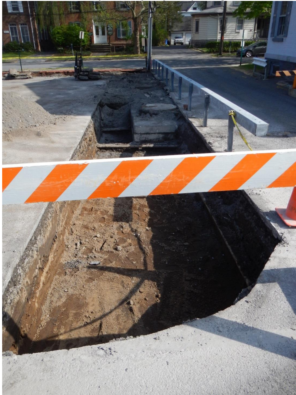
Removal of material from future planting bed
