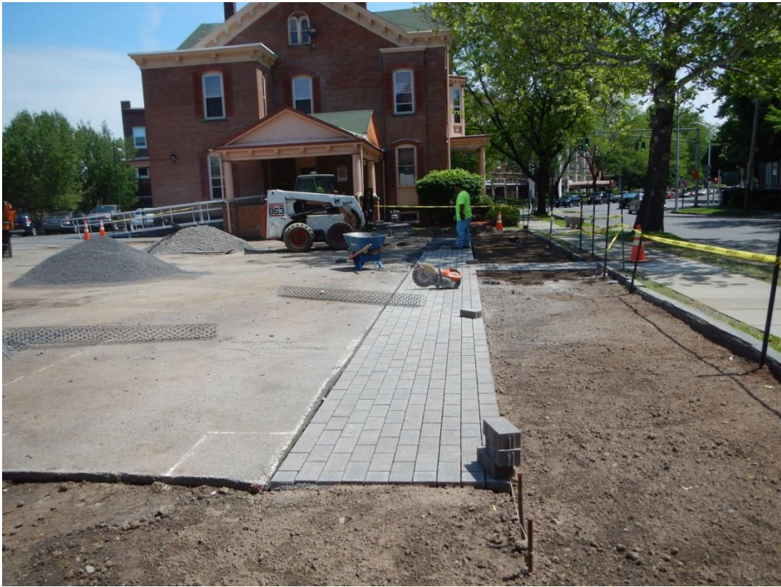
Completed installation of the permeable pavers
