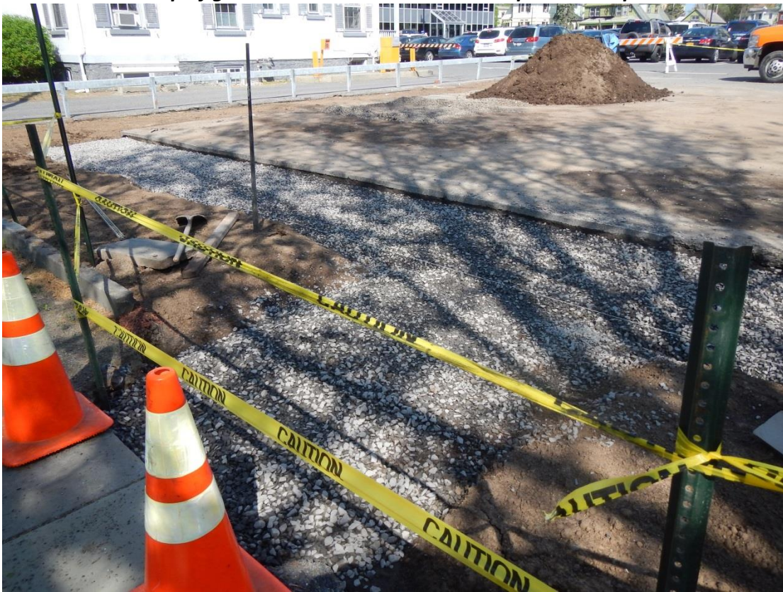
Close-up of gravel sub-base underneath the permeable pavers
