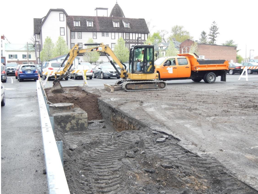
Replacement of existing fill (bottom) with the bioretention soil mix (top)
