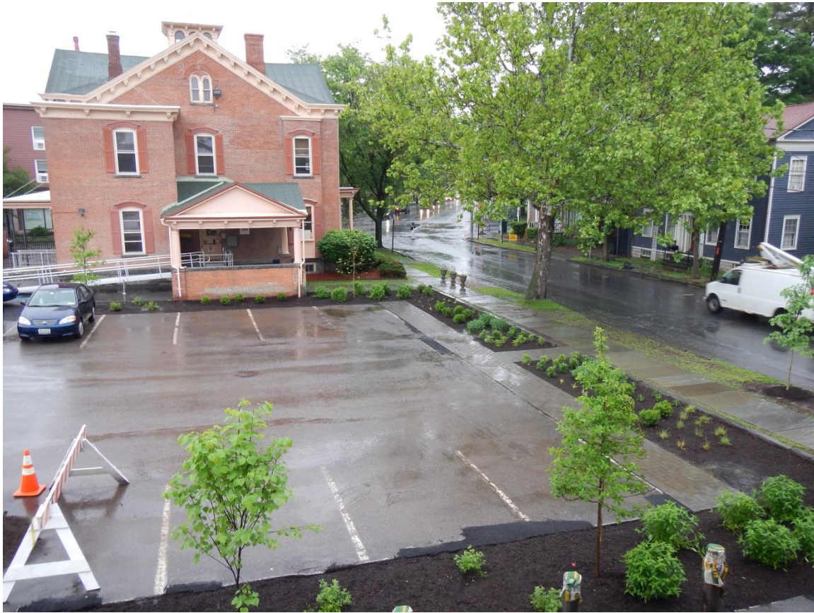
Bio-Retention Area during a rain storm (6/5/14)
