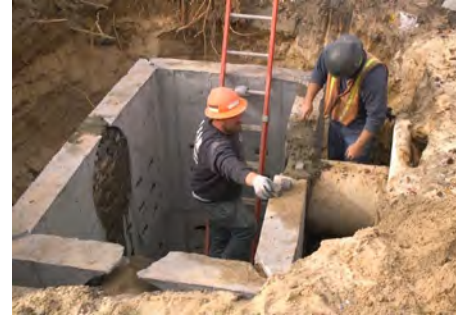
Workers installing vortechs stormwater basins on Roanoke Avenue, Riverhead Photo: CCE
