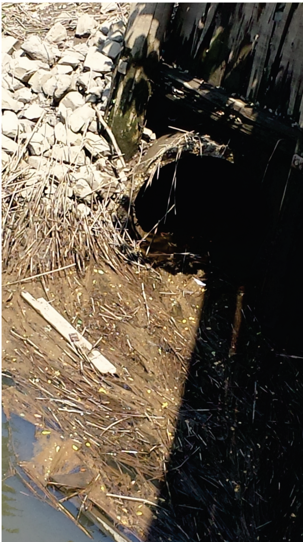
Picture 2 : Possible pollution source- outflow pipe at site M3 (Matawan Creek), July 2014. The pipe is only visible at low tide.
