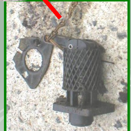
Leaking Drain Valve
