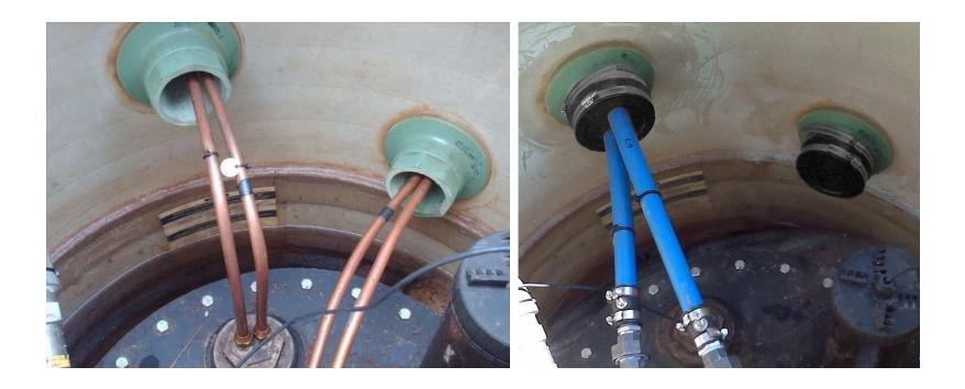
This split repair fitting design starts with a center ring sized to the pipe or conduit. The outer ring is applied over the center ring and a band clamp is tightened around the assembly.
