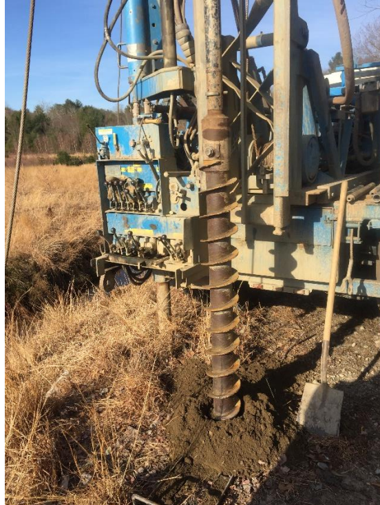
Boring auger digging first soil bore. Soil bores were dug to approximately 20 ft, or if bedrock was hit, which ever came first.
