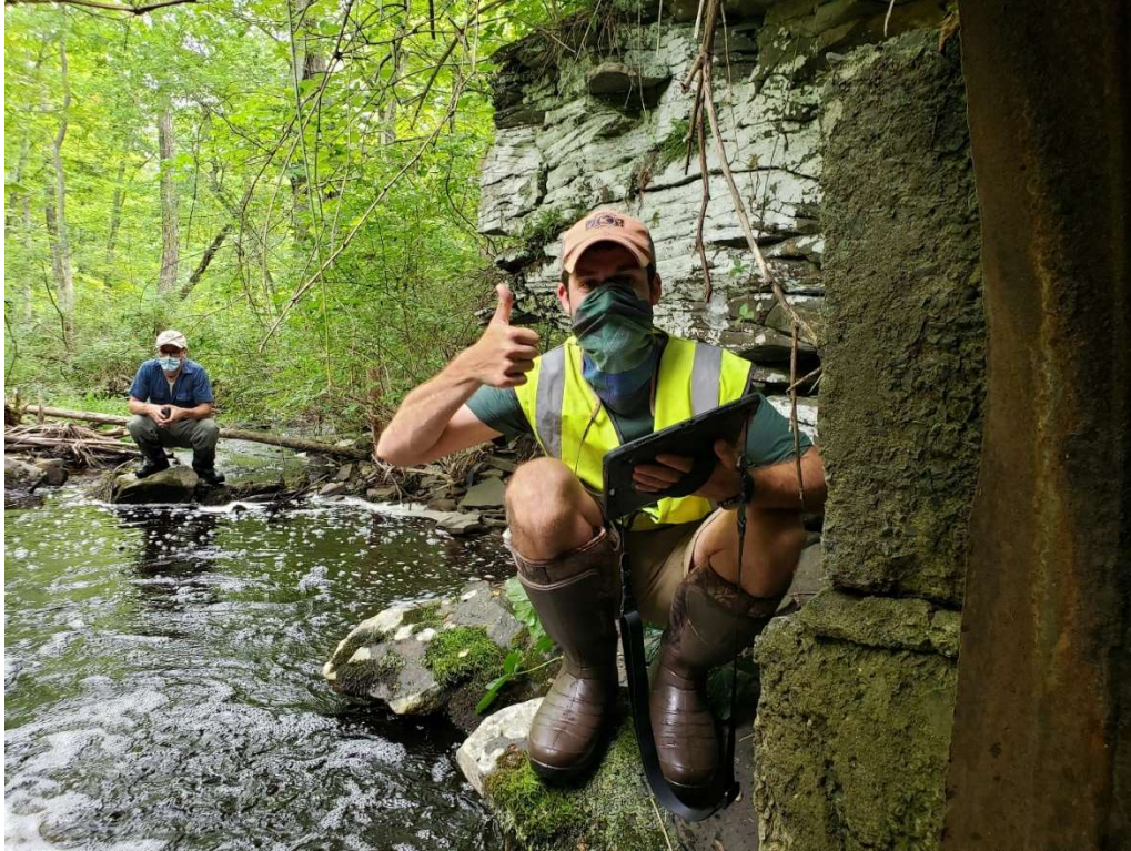
Tim and Ben on the outside of an impressive downstream scour pool.
