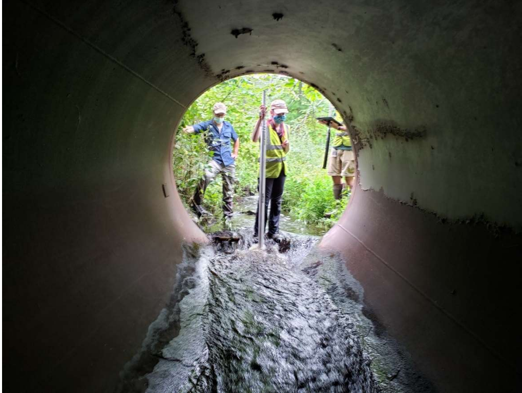
Tim, Ben, and Kiah standing at the inlet of a round culvert. Measurements are being taken using a stadia rod and an iPad. Tim is standing on failed upstream armoring that has channelized the stream.
