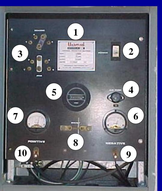
1. Data Plate 2. On/Off Switch 3. Tap Settings 4. Fuse 5. Hour Meter 6. Amperage 7. Voltage 8. Shunt 9. Negative 10. Positive
