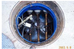
Transition/intermediate sump:
