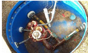
Sump sensor in contained turbine sump
