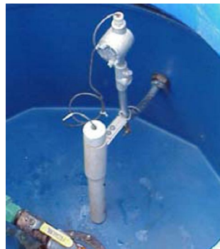
Float Sump Sensor:
