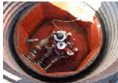
Contained turbine sump:
