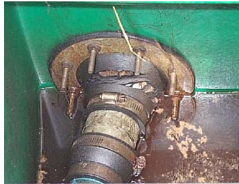
Seals in poor condition
