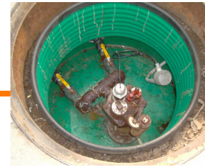
Uncontained turbine sump:
