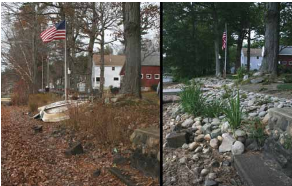
Before and after pictures of the Attitash shoreland protection project. (Left) Note the rock stains of the normal summer water level mark in the lower right corner. (Right) Native shoreland plants and natural indigenous stone overlying erosion-protective filter fabric will stabilize the previously eroding shoreline, provide important lakeshore habitat, and enhance aesthetics and property values.
