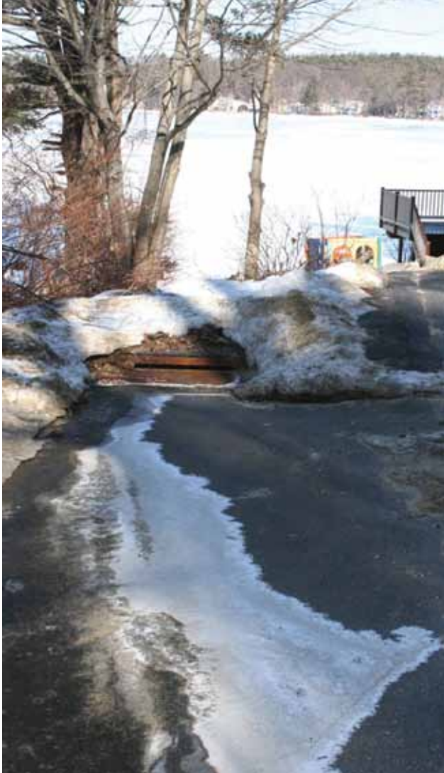
A storm drain conveying road salts and fine sediments into Lake Attitash.
