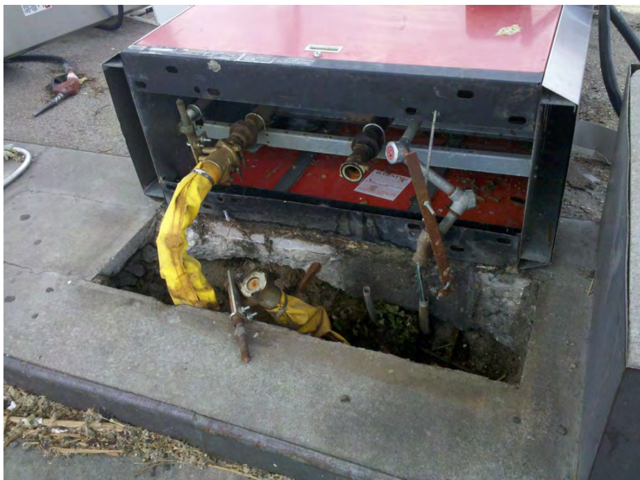
"The Store" sustained only minor tornado damage, but the fiberglass piping was broken when the dispensers were blown over.
