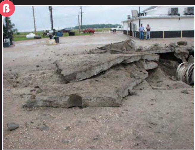
B Two large concrete slabs from the top of the diesel tank were blown up and landed upside down on top of each other.
