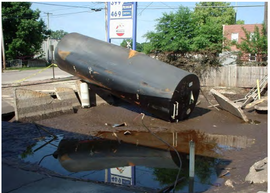
Clark station tank that floated out of the tank pit. The site was covered by seven feet of water.
