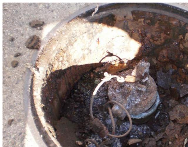
Top: Typical ATG riser installation surrounded by the tank backfill. Overflow events can leak from such unprotected risers and spill directly into the tank backfill. Such releases can be prevented by locating all risers within a collared sump.
