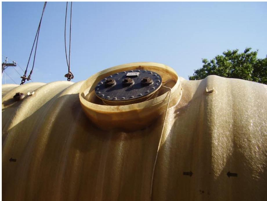
*A tank equipped with a collar for attaching a full-depth sump. Such collared sumps provide secondary containment and can be used to isolate tank risers and spill buckets from the tank backfill material.*
