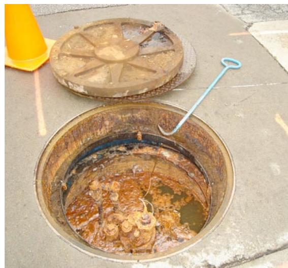
STP sump showing biological mat from a 2008 inspection at an E10 facility.
