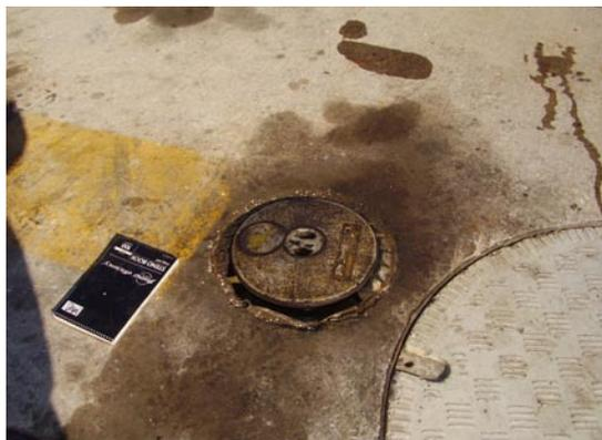
*Damage to a spill-bucket support ring. Such damage allows surface spills to enter the tank backfill.*
