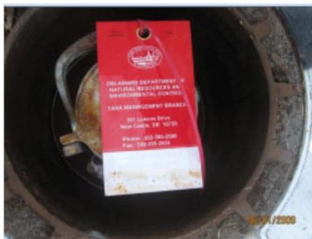
FIGURE 1. Red tag on fill pipe in Delaware.
