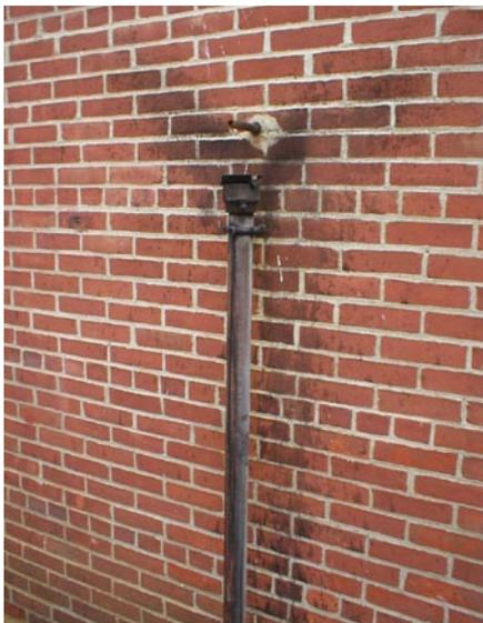
*Product was released from the vent cap during an overfill event. A leak in the single-walled vent line resulting from improper installation, corrosion, or movement of the vent riser would result in a product release into the backfill during such an overfill event. Gasoline vapors and vapor condensates can also be released from these leaking vent lines*
