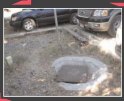
This installation contractor must have run out of concrete while pouring the form for this custom-made sump. Or was this intentional so the square lid would fit over the round sump?
