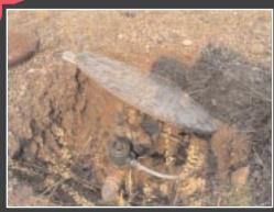
Note the beautiful grain on this craftsmanstyle, custom-built plywood sump lid. Also note its water-tight seal to the sump walls.
