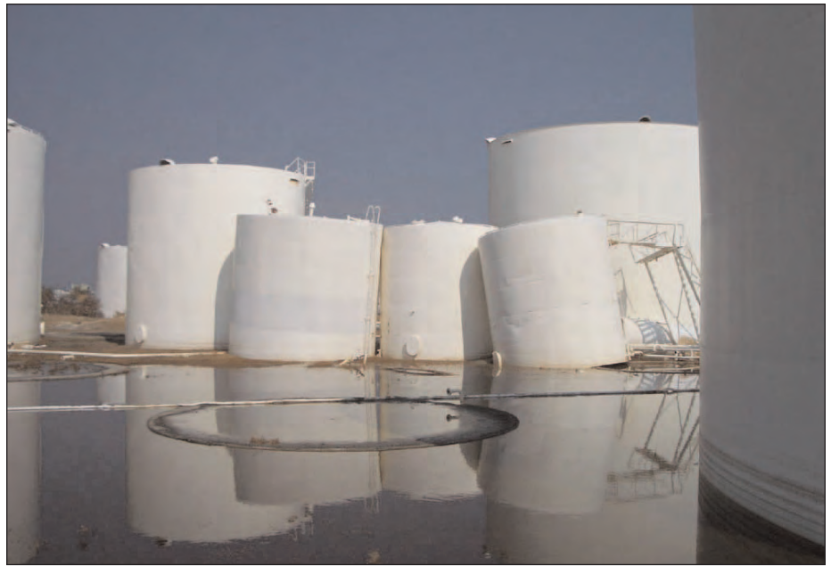
The ASTs at this Munroe Barge Terminal in Biloxi floated off their footings. A release of 482,000 gallons of fuel occurred, but no evidence of this fuel was ever seen (presumed "lost" out to sea). The three tanks that floated up against the larger tanks are 75,000-gallon gasoline tanks.
