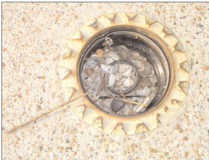
Cap gone from tank fill allowing four-inch riser to become filled with sand and debris during storm surge. This tank was found to be completely full of water with nine inches of sand/debris in the bottom.
