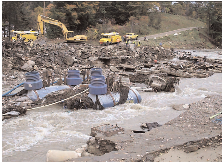
The facility just after the river rerouted through it. Only the tanks remain; the building was washed away during the flood.
