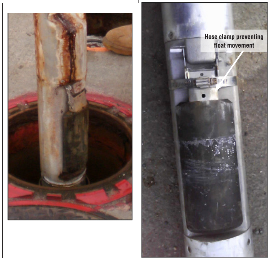
Figure 3. Movable floats on drop tube shutoff devices may not move. This may be due to corrosion (left photo) or human interference (right photo). Photos courtesy of Spruce Wheelock.
