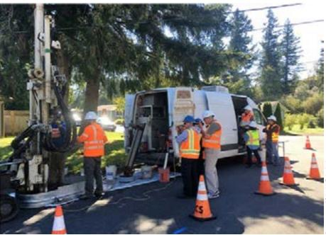
An example of a direct-push drilling rig coupled with a direct-sensing van during the process of conducting a real-time high-resolution site characterization. The small, versatile footprint of the units allows for easy maneuvering at sites. The clean direct-push drilling approach virtually eliminates costly waste-handling requirements."
