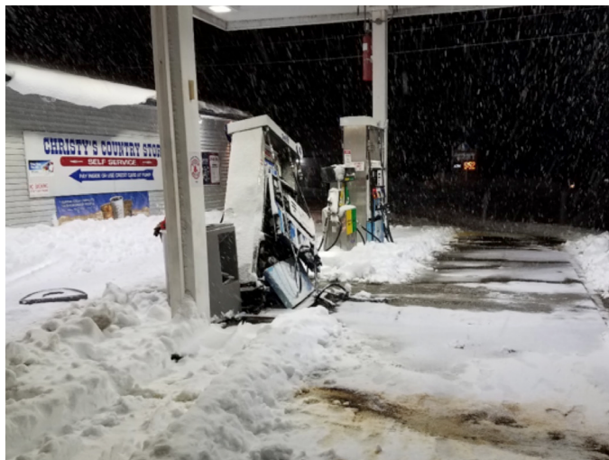
Dispenser when it was found by the fire department. Notice the streams of fuel.
