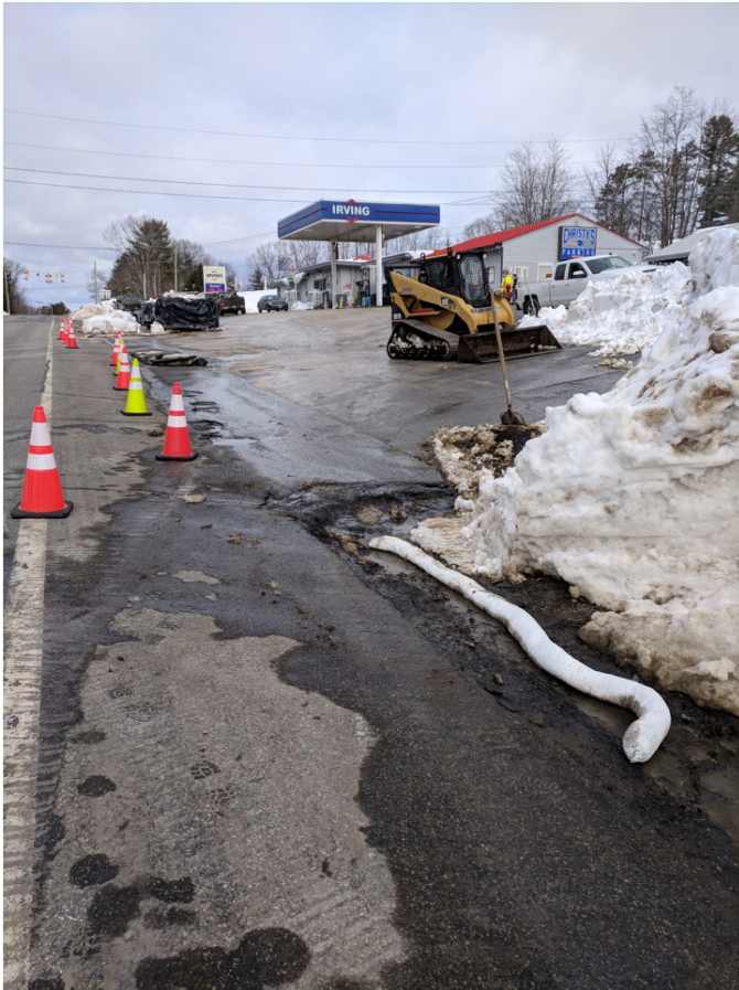
Contaminated snow removal a day after the spill
