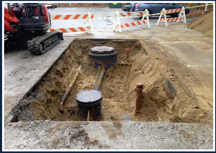
Single-walled components often leak for long periods of time before detection.
