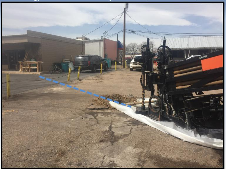
Remedial Strategy: 2 Parallel Horizontal Injection Wells, 3-inch Diameter, 21 feet BGS
