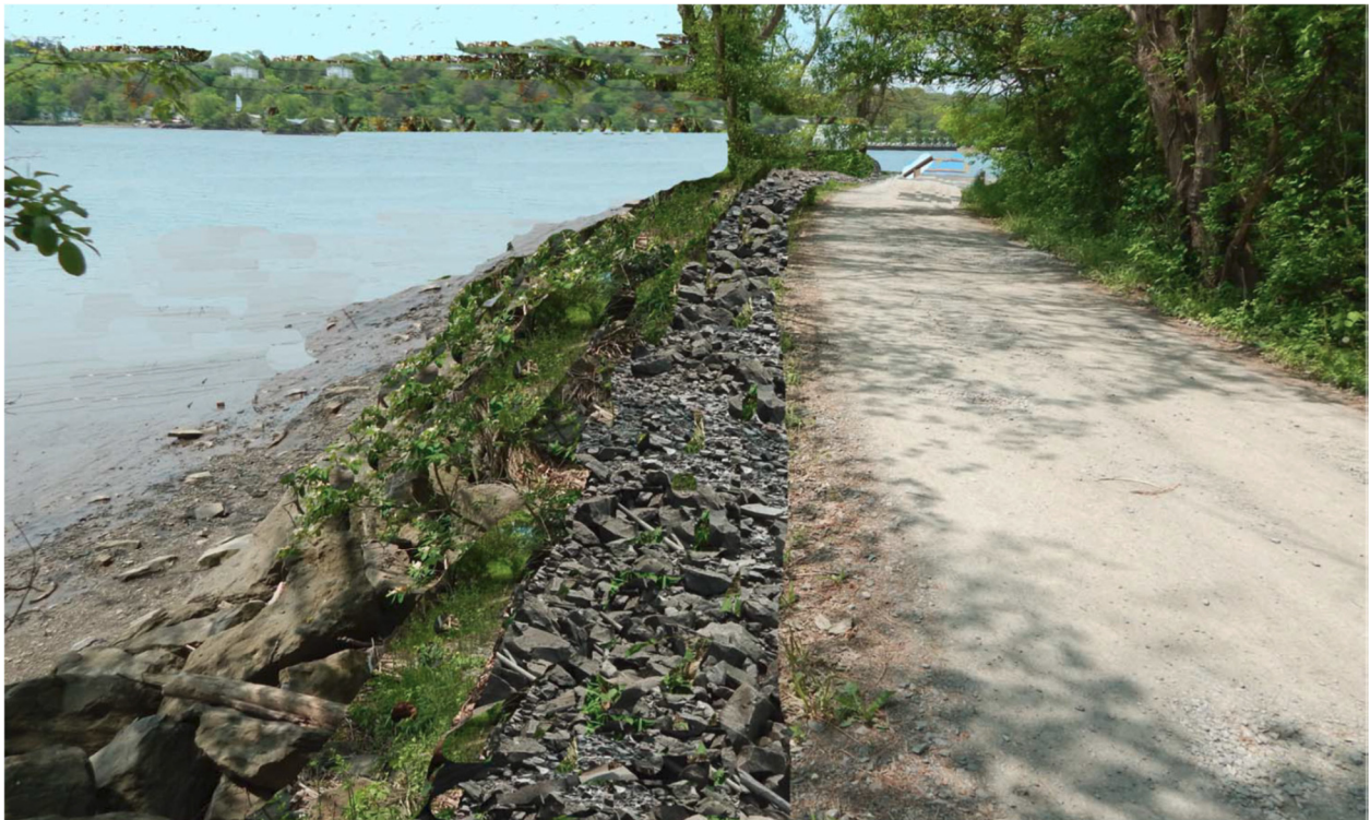
Photo 2. Visualization of road base armor (using stones and grasses)
