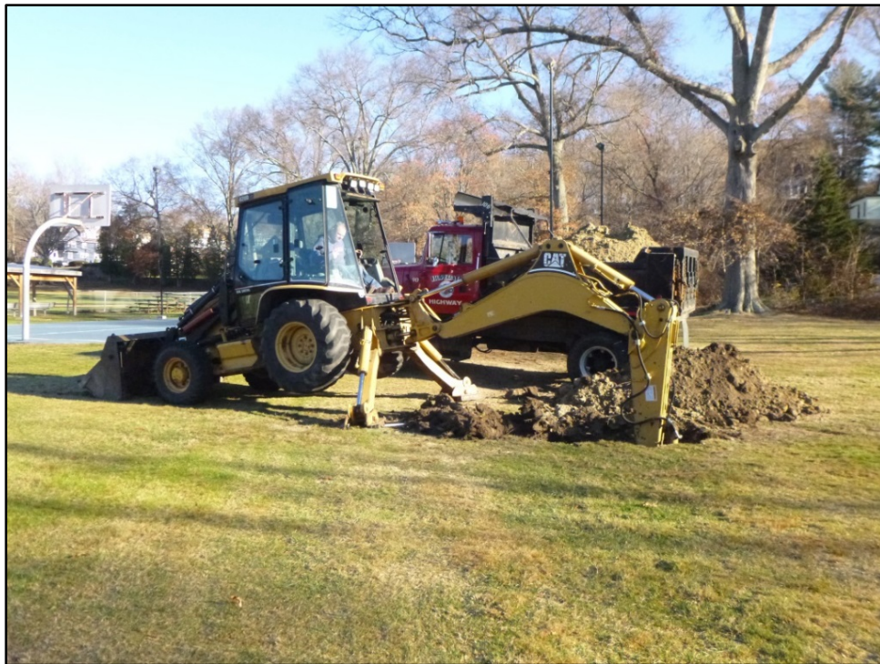
Figure 7—Excavation of the soil test pit.
