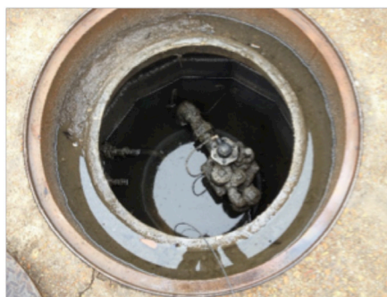
Figure 1. Typical “old” containment sump that stays full of water and does not serve as secondary containment.
