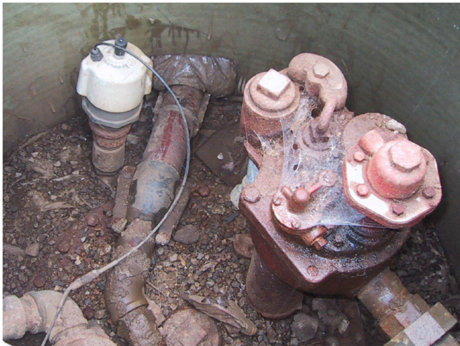
Figure 1. Early versions of double-walled piping were only concerned with containing the pipe. In the photograph above, 2-inch diameter primary piping was installed inside 4-inch diameter secondary piping. A 4 x 2-inch reducing fitting was used to seal off the interstitial space of the pipe. There was an opening in the bottom half of the reducing-fitting (not visible in the photo above) where a sensor could be installed. On this tank, the opening on the bottom of the reducing-fitting was left open, and leak detection consisted of an external leak sensor located under the white cap at the upper left. Note the primitive penetration fitting where the piping comes through the wall of the manhole.
