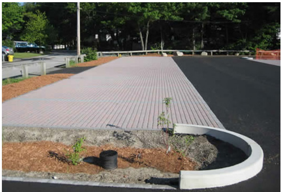
Pervious paving and bioretention in a parking lot – credit: Mass.gov
