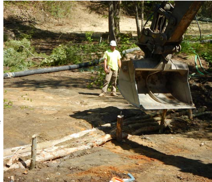
Crib wall construction, McQuesten Brook, Bedford, NH – credit: NHDES Staff
