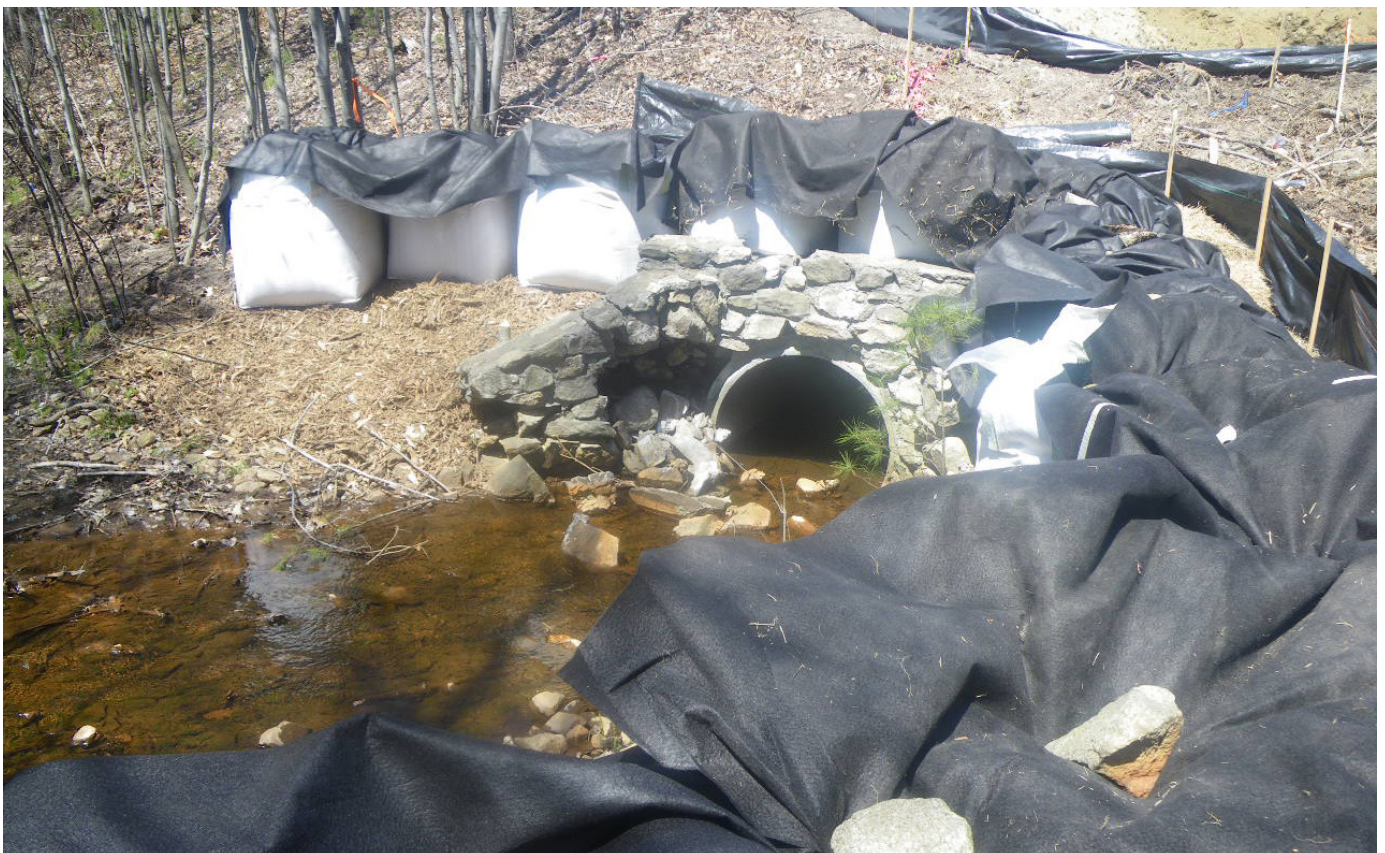
Erosion and sedimentation controls – credit: NHDES Staff
