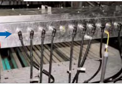
$Arrow\ indicates\ high-water\ mark\ on\ the\ Keene\ plant's\ UV\ equipment.$
