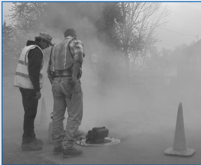
After injecting smoke into a sewer in Ravena, N.Y., observers monitor where the smoke emerges; inappropriate releases can indicate illicit connections, line punctures, or faulty pipes. Periodic smoke testing of a collection system is part of an effective CMOM program.
