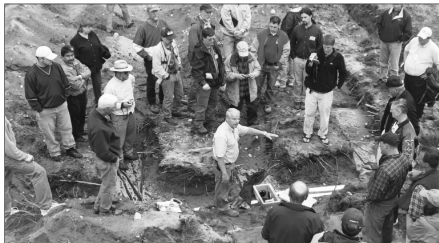
George Barden, Ontario County (N.Y.) Soil and Water Conservation District, leads conference participants through the process of installing an onsite wastewater system at a new residential development.
