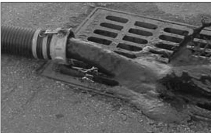
Sludge consistency can vary from a low percent solids (L) to a high percent solids (R).
